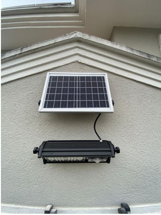
Figure 1 | Actual product installation
